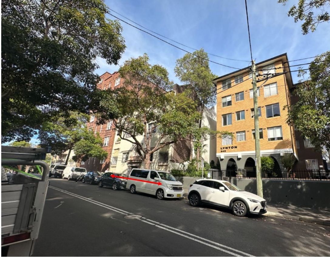
front of site looking south-east along Liverpool Street
