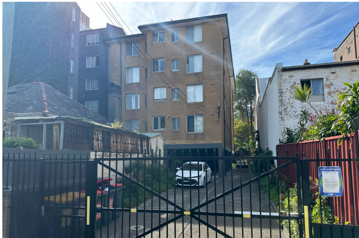
Looking north towards the rear setback of 349 Liverpool Street and the heritage item cottage of 1 Darley Place to the left
