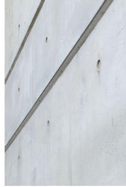
OFF FORM CONCRETE
